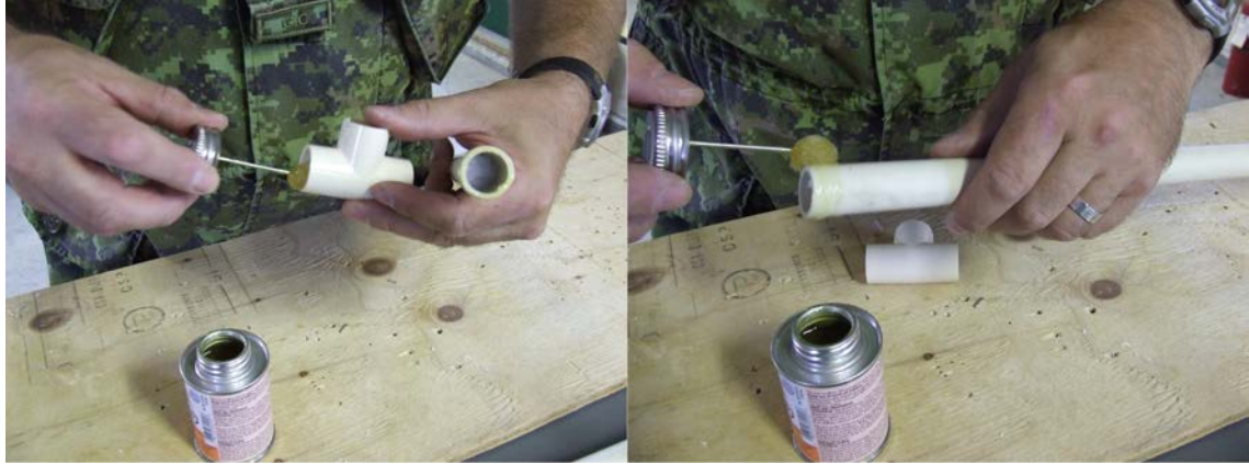
Figure A-6 Applying cleaner or glue to the joint surfaces before gluing.
